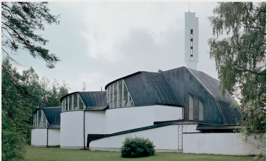
"Church of the Three Crosses": the partition of the eastern façade
